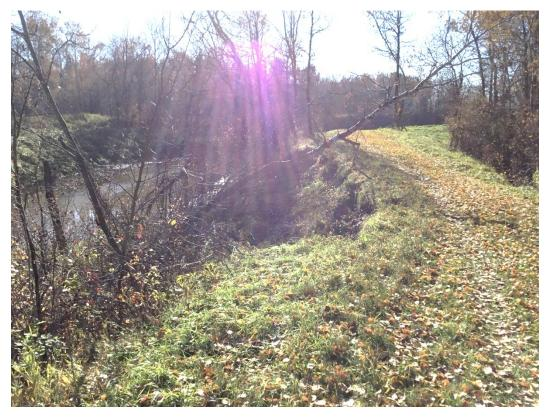
Judicial Ditch 23 outlet stabilization construction was nearly completed, though some touch-up work (slopes were let in rough shape) and buffer planting must still be completed (in the spring or summer of 2022). In addition to the rock structures at the outlet of the ditch, the last 0.6 miles of the ditch were resloped and two side water inlets were installed.
